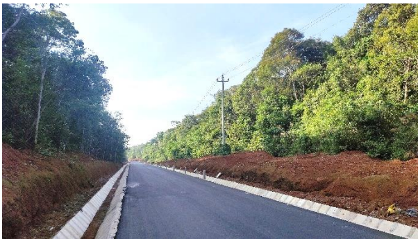
Newly paved road
